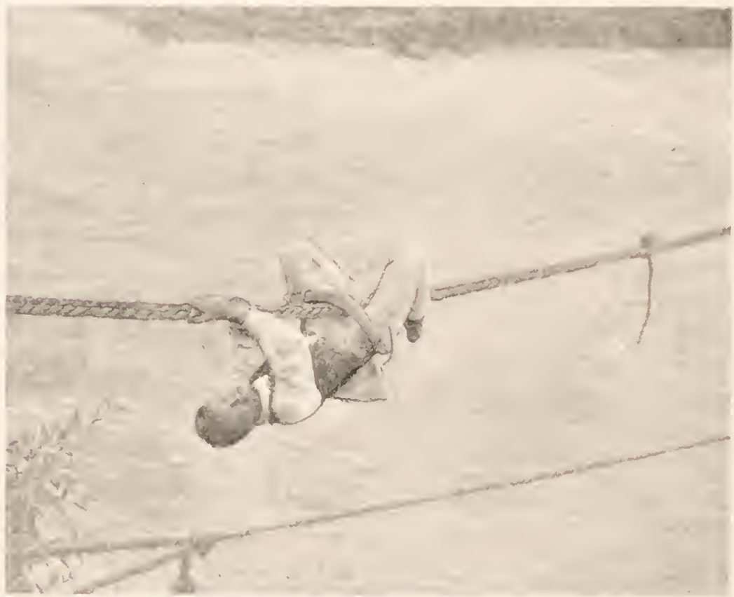
NATIVE CROSSING ROPE BRIDGE
